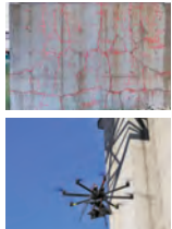
Inspection applying photographic technology (by our own UAV)
