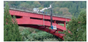
Inspection by our own bridge inspection vehicle
