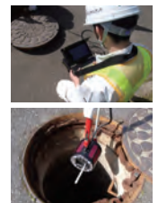
Inspection by pipe opening camera
